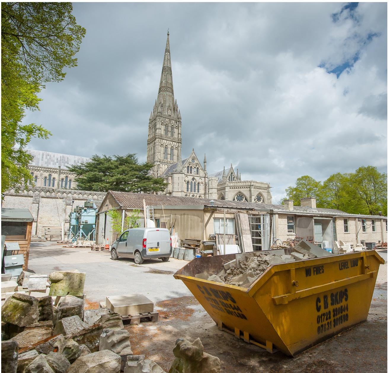
Image 6: The existing Works Department
